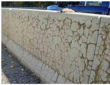
Fig 1. Effects of Alkali-Silica reaction
