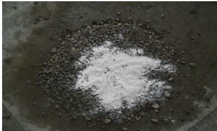
Mixing of fibre and metakoalin in concrete.
