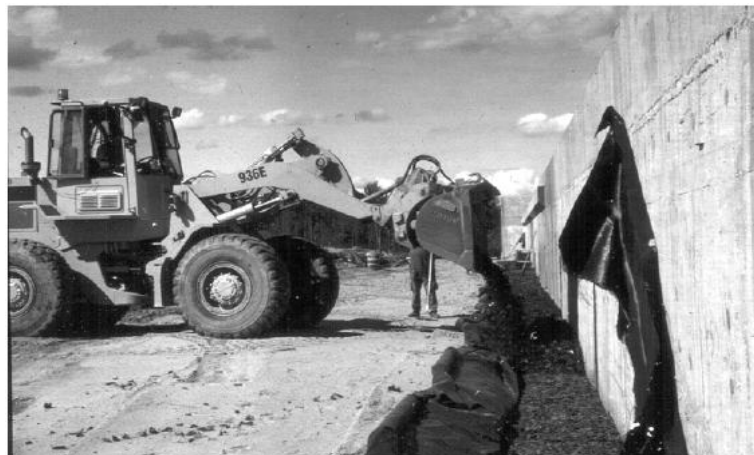
Figure 3.2.2 Placing Tyre Shreds using Front End Loader for Rigid Frame Bridge
