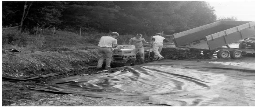
Figure 3.3.2 Placing and Compacting Tyre Shreds in Edge Drain
