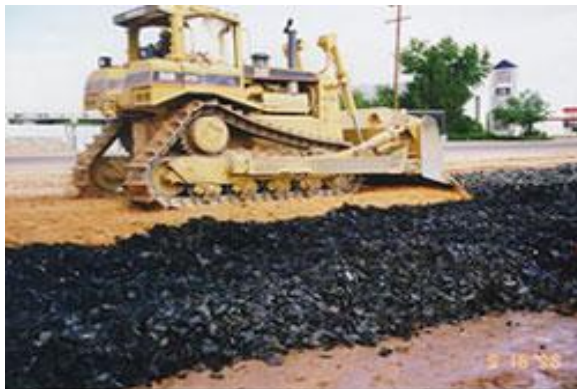
Figure 3.1.2 Road Embankment constructed with Shredded Tyres
