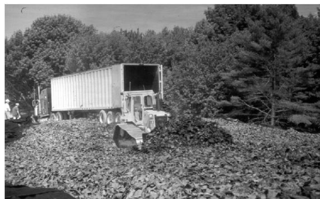
Figure 3.1.3 Caterpillar D-4 Spreading Tyre Shreds for Lightweight Embankment Fill
