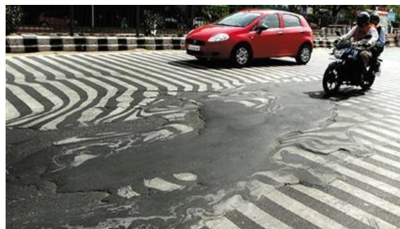
Fig1. A section melted pitch surface of a road near a hospital in New Delhi and its deformed zebra lines [3] .
