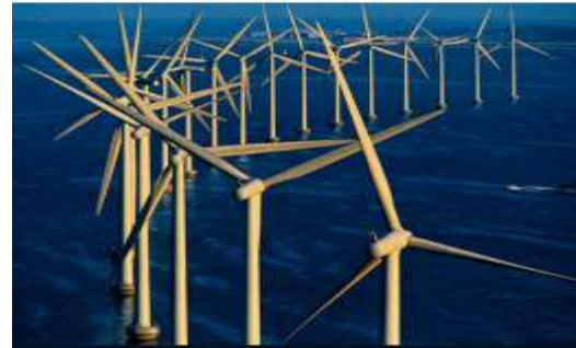
Fig2.12. Offshore wind farm (Source: www.google.com)
