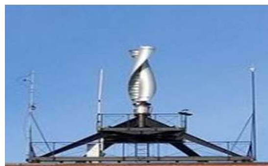
Fig2.10. A twisted Savonius wind turbine(Source: Wikipedia)
