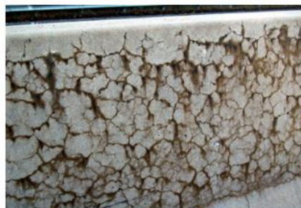
Fig3. Deprivation by the aggregate development paving the way to the further concrete deprivation (Zoran Bonić, Gordana Topličić Ćurčić, et al. 2015).
