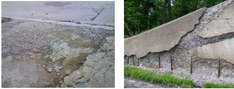
Fig4. Concrete degradation caused by crystallization of road defrosting salt (Zoran Bonić, Gordana Topličić Ćurčić, et al. 2015).
