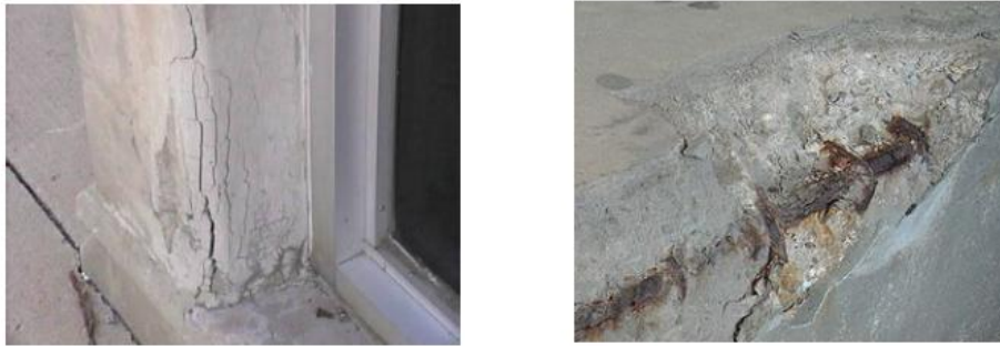
Fig5. Concrete carbonation paved the system for frost accomplishment (Zoran Bonić, Gordana Topličić Ćurčić, et al. 2015).
