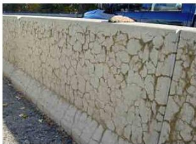
Fig3. Deprivation by the aggregate development paving the way to the further concrete deprivation (Zoran Bonić, Gordana Topličić Ćurčić, et al. 2015).
